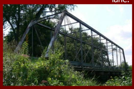
Project scheduled to start summer 2015 and finish in the spring of 2016. Construction process would include disassembling structure and repairing and/or replacing truss members. All truss members will be galvanized and existing stone abutments will be repaired. The current deck may be replaced with a reinforced polymer deck.
