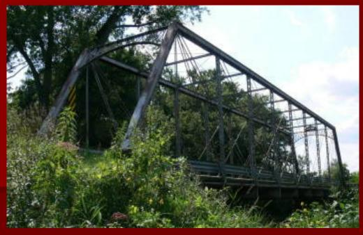
Project scheduled to start summer 2015 and finish in the spring of 2016. Road improvements would currently be scheduled for 2017. Construction process would include disassembling structure and repairing and/or replacing truss members. All truss members will be galvanized and existing stone abutments will be repaired. The current deck may be replaced with a reinforced polymer deck.
