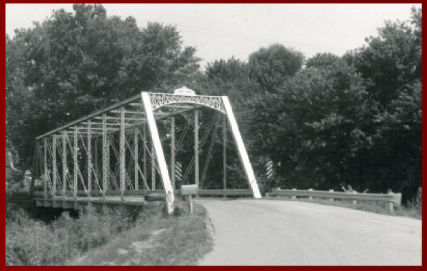
Built in 1882 by the Massillon Bridge Company, the current bridge has high historical significance. It's a technologically significant bridge type as this Whipple truss bridge is an example of the double-intersection Pratt thru truss bridges that were very popular in the 1880s. In addition, this bridge is eligible for the National Register of Historic Places.
